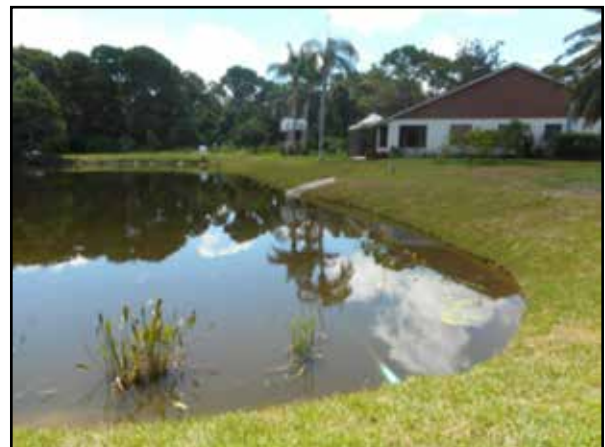
Completed shoreline with remediation and aquatic plantings
