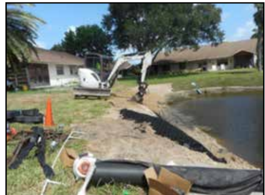
Installing the Geoweb process.
